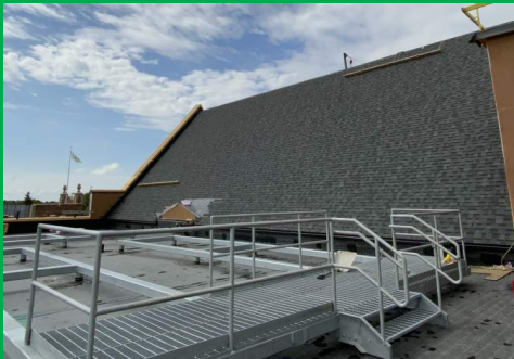
EAST FACING SLOPED ROOF
