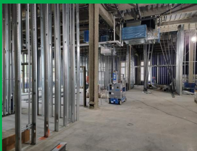
LEVEL 1 - NORTH EAST CORNER
