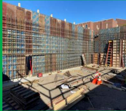
Foundation Wall Forming and Rebar
