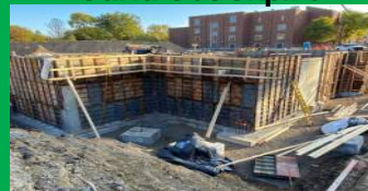
Poured Foundation Wall
