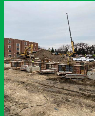
North Foundation Wall Forming
