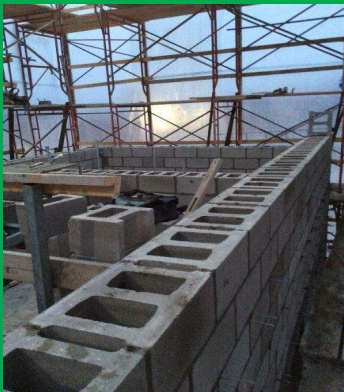
South Stair/Elevator CMU Erection
