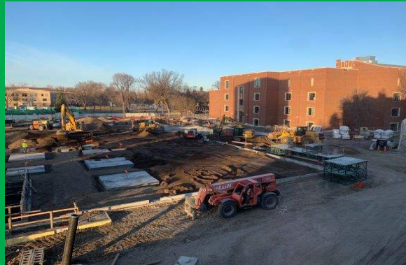
South Footing and Foundations
