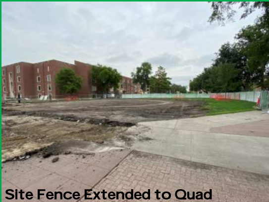
Excavation For Soil Correction
