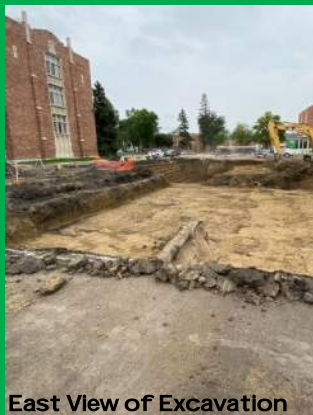
East View of Excavation
