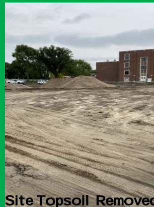
Excavation For Soil Correction
