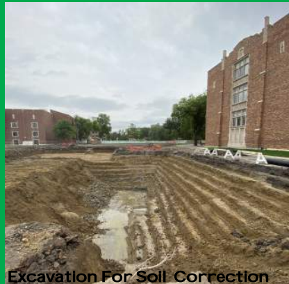
Excavation For Soil Correction
