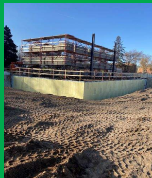
South Elevator and Stairwell
