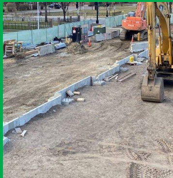
West Wall Backfilled
