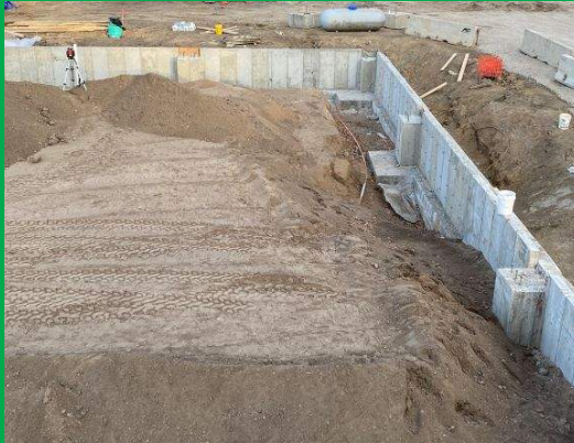
Foundation Wall Backfilling
