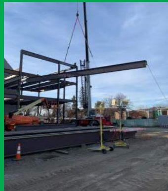
Steel Erection
