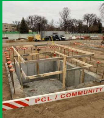
North Elevator Pit
