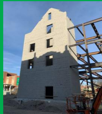
South CMU Stairwell and Elevator Shaft
