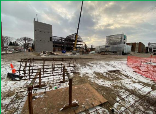
North - East View of Site
