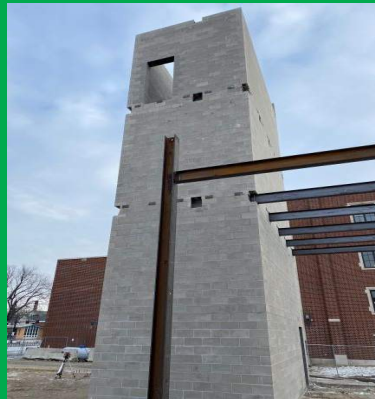
East CMU Stairwell
