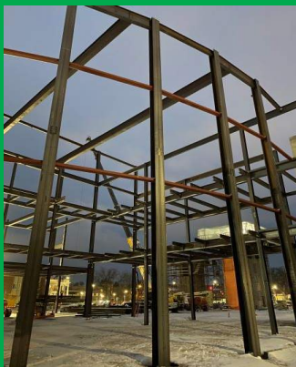
Curtain Wall Steel
