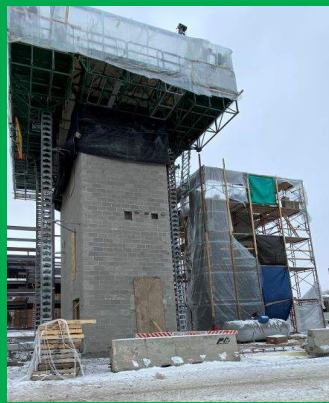
North CMU Stair and Elevator
