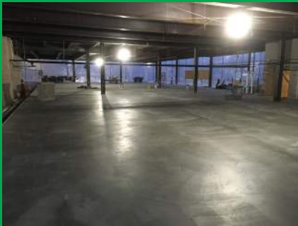
Level 2 Slab on Metal Deck
