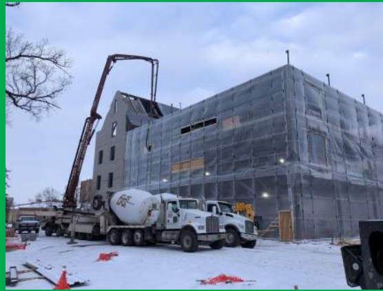
Pump Truck Pouring Concrete
