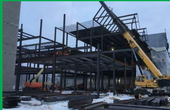
Sequence 3B Structural Steel Framing
