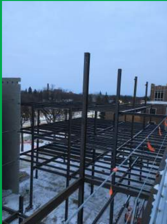
Sequence 3A Structural Steel Framing
