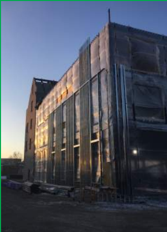
Metal Stud Framing on South Elevation
