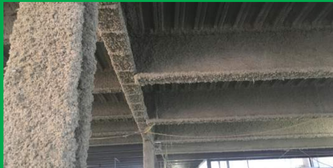
Fire Proofing of Structural Steel
