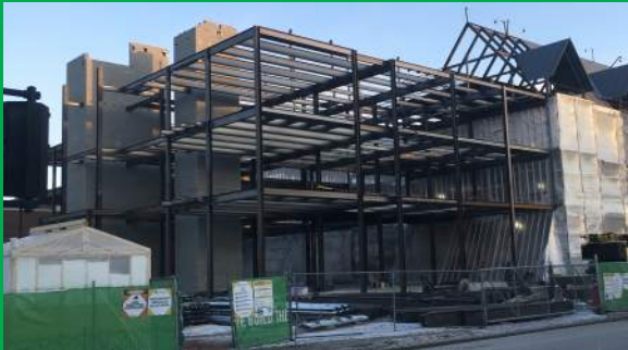
North West View of Building
