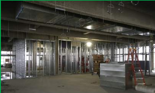
Interior Metal Framing Level 3
