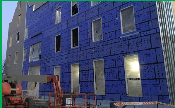
South elevation prepped for air barrier
