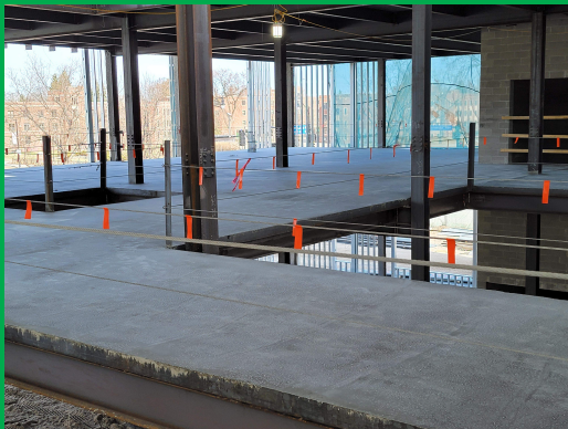
Sequence 3 Level 2 slab on deck
