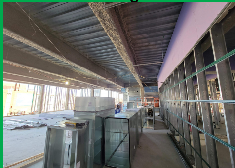
Sequence 2 Duct main installation
