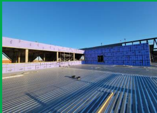
sequence 2 low roof framing/sheathing
