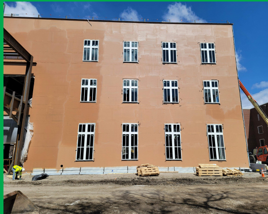
South side windows and air barrier
