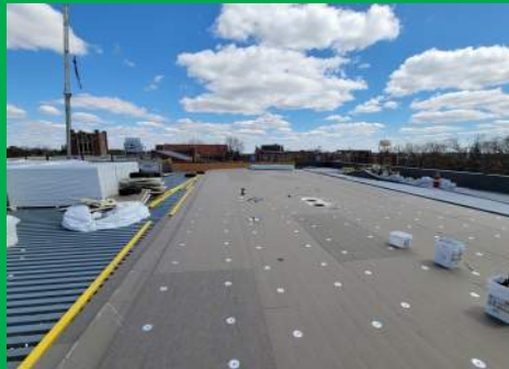
Sequence 1 Low Roof Installation
