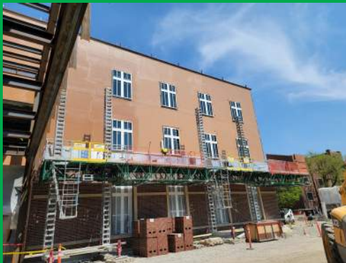
SEQUENCE 1 SOUTH WALL BRICK INSTALLATION
