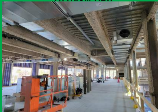
LEVEL 2 SEQUENCE 2 DUCT MAINS
