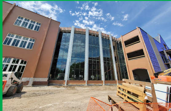
CURTAIN WALL INSTALLATION
