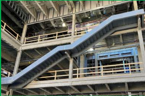
CENTER STAIR FROM 2ND TO 3RD FLOOR
