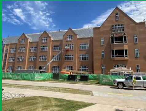
SOUTHEAST ELEVATION MASONRY
